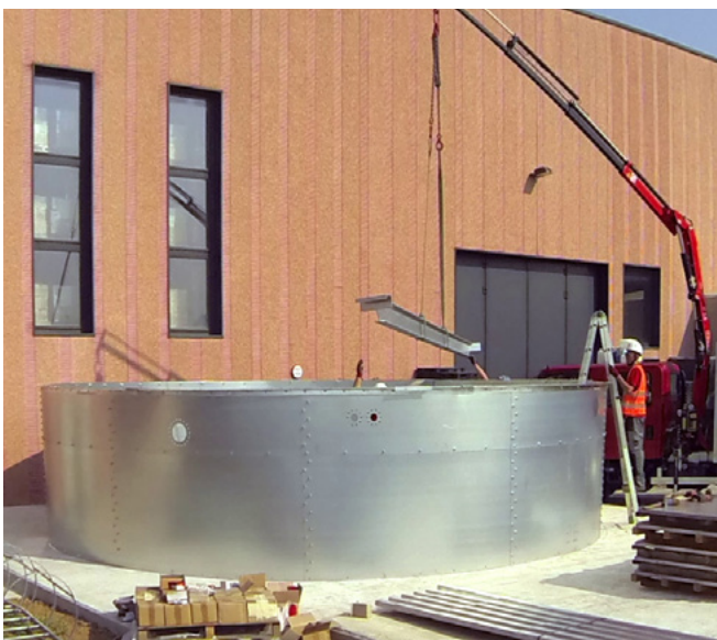
Installation of roof beams
