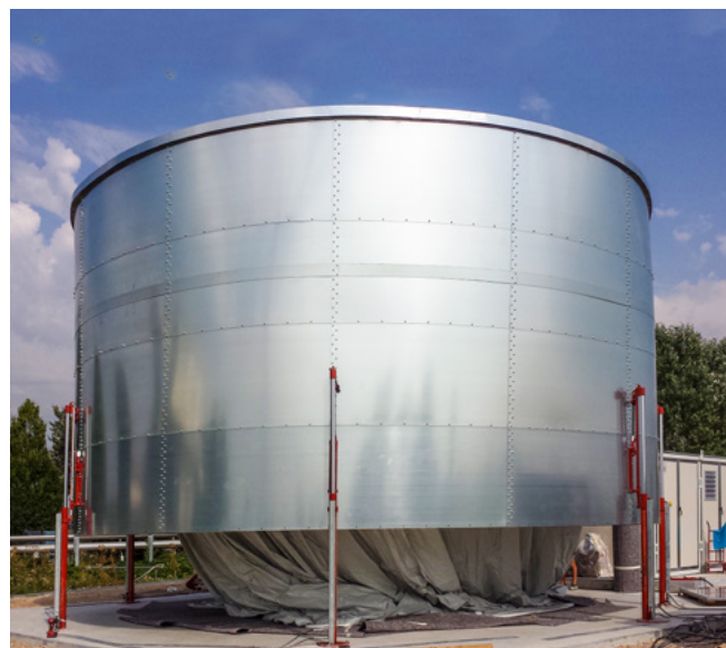
Tank installation with jacks
